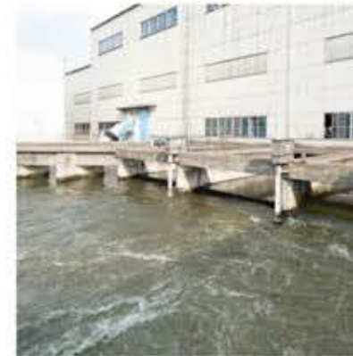
3,100 m 3 testing tank
