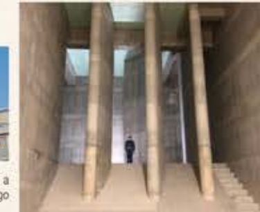
▲ The New Large Pump Production Building, which houses a large, 3,500 m 3 testing tank that's 11 m deep, at the Yonago Plant at the time of completion
